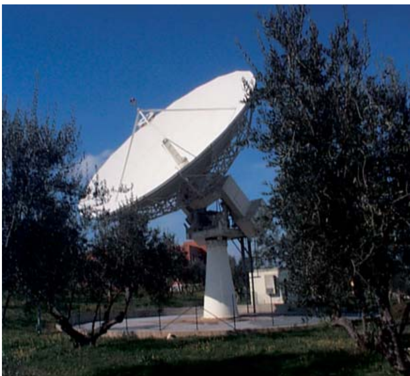
Figure 3. The User Earth Terminal reception antenna at ESRIN, for Envisat data acquisition via Artemis
